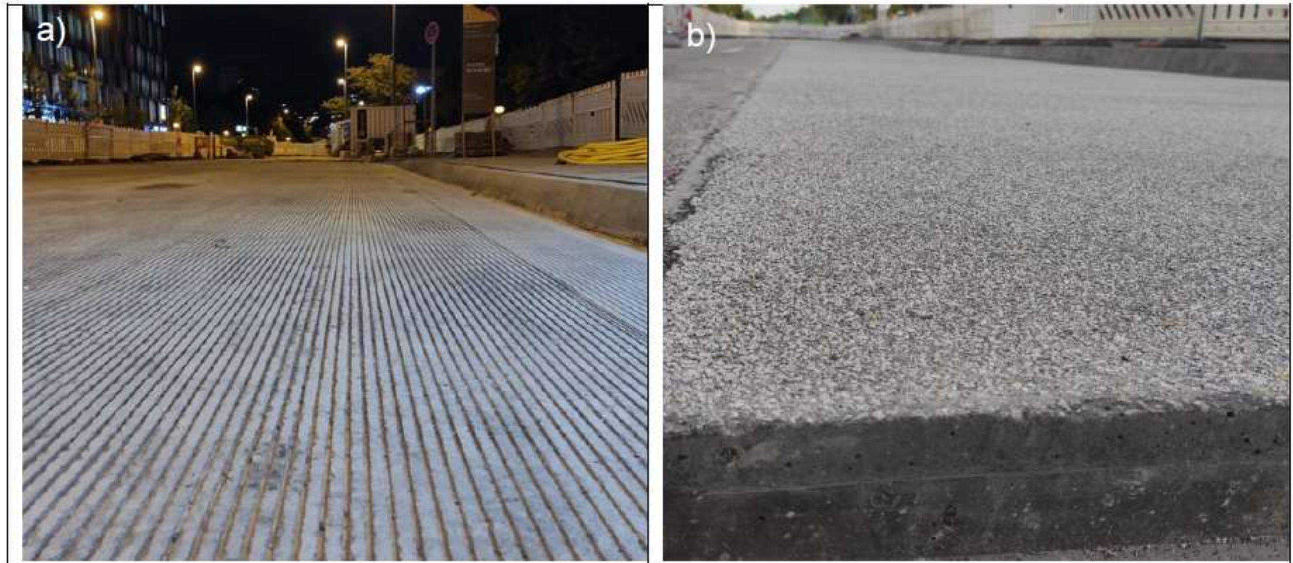
Figure 3: Surface preparation by a) grinding and grooving and b) chipping-matrix
